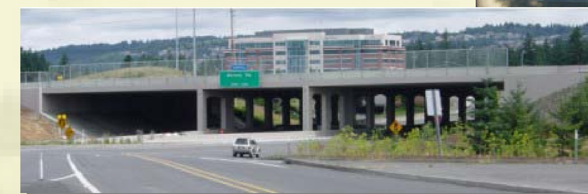
Precast Slab Bridge on Hwy. 26
