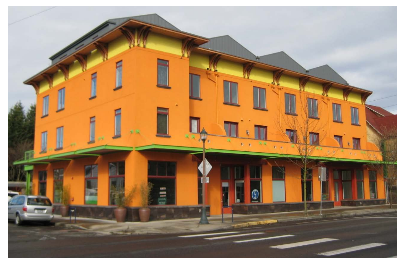
(C) Building constructed with ICF grid walls
